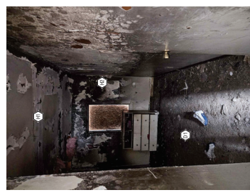
B VIEW OF GYPSUM BOARD - BEDROOM 1
